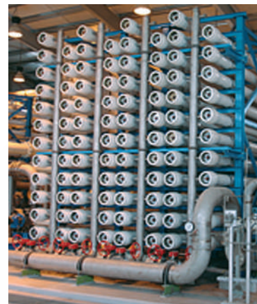
SWRO train with HPB at lower right
