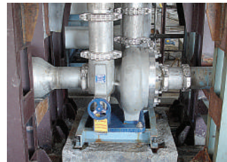
Retrofit installation at a power station in India
