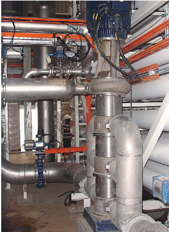
LPH with 3 modules in Singapore
